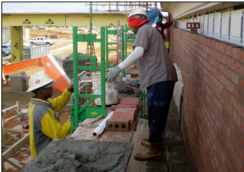
Bricklayers topping out a 14-foot-high brick veneer.
