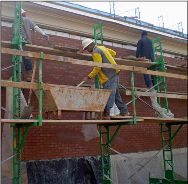
Land tubs of mortar, full pallets of block, or 400 brick on the Laborers' Platform. WORKHORSE can take it. 3,800 pounds per bay max. (Never exceed the capacity of your planks.)
